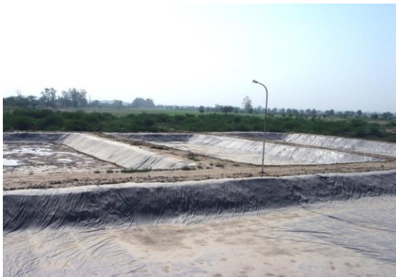
Figure 1: Poly-lined ponds to reduce the seepage loss
